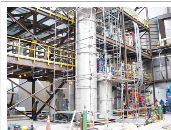
Tri-State is participating in chilled ammonia post-combustion carbon capture pilot plant presently being tested at the WE Energies Pleasant Prairie Power Plant in Wisconsin.
